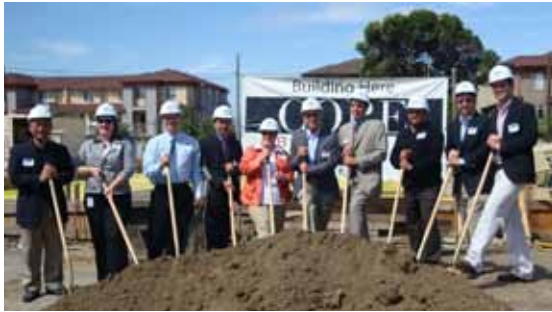
Core Companies' executive team, public officials, city staff and project financiers break ground on Cornerstone project.
